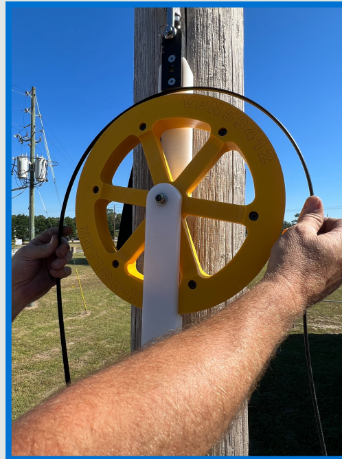
Place cable onto wheel
