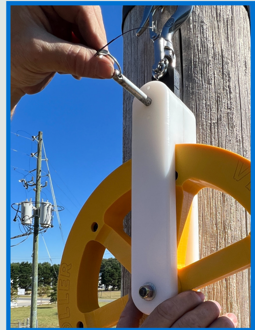
Re-insert retainer pin
