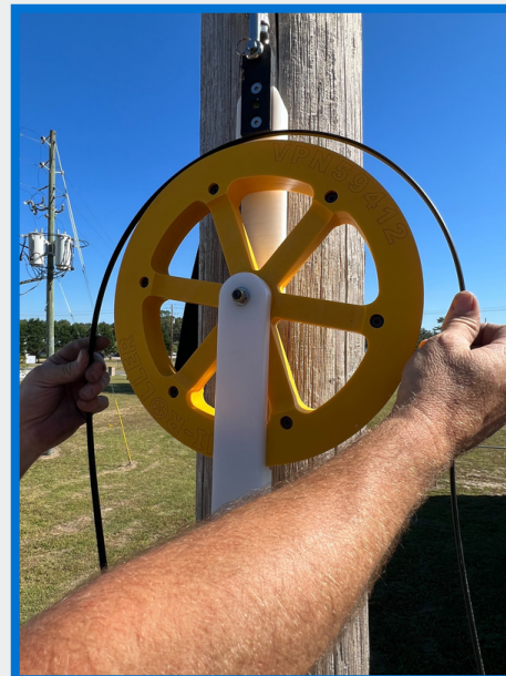
Place cable onto wheel
