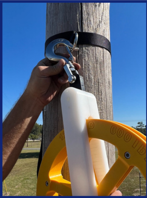
Attach Hi-Roller to existing pole line hardware or pole strap (VPN 59401)
