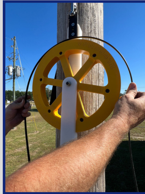
Place cable onto wheel
