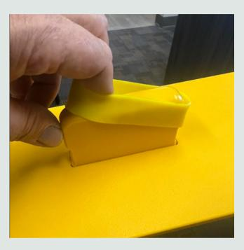
Wrap Silicone band around Fin from the bottom side and position band into groove.
