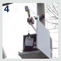
Using cordless drill in the forward direction, press the drill trigger to raise payload to the desired position.
