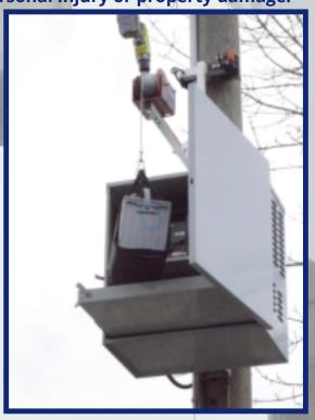
cinching straps. The rubber mounting brackets attached to the hoist frame have been designed using the profile specifications of many of the most commonly used utility poles. They are also capable of supporting the load in all kinds of weather conditions.
