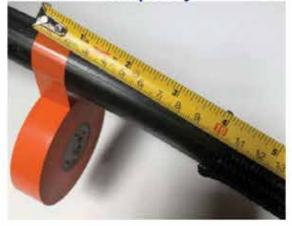
Continue wrapping an additional 4 inches of tape onto the mesh, pulling tightly until the mesh pattern is visable.
