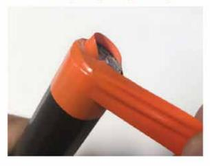
Begin wrapping tape onto cable 4 inches below the mesh.
